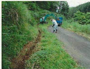
側溝掘削100m
